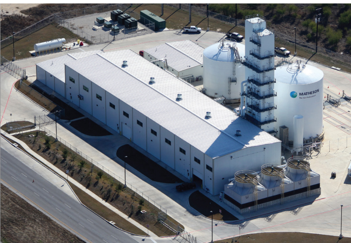
Nippon Sanso Matheson Air Separation Unit, San Antonio, TX
